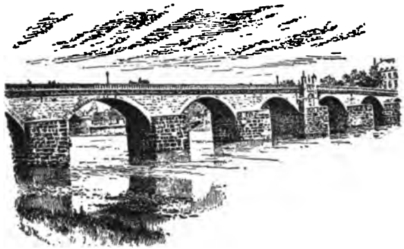
OLD ROMAN BRIDGE OVER THE MOSELLE, GERMANY
